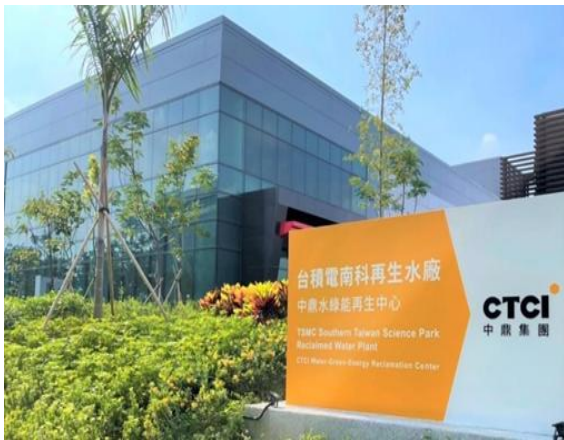
TSMC Southern Taiwan Science Park Reclaimed Water Plant
